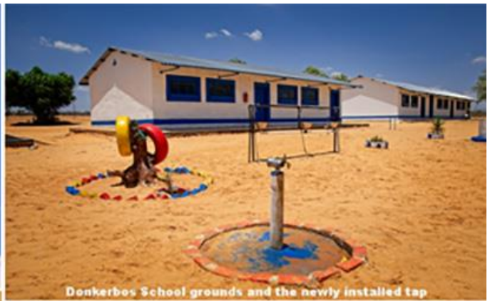
Donkerbos School grounds and the newly installed tap
